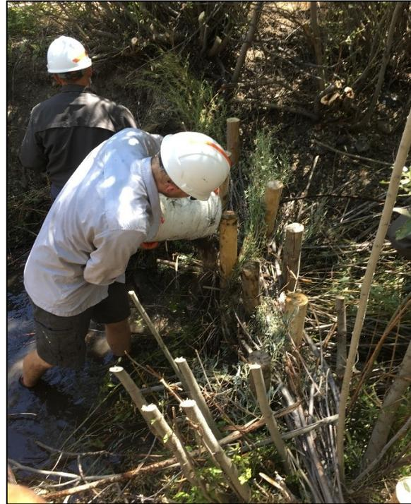
*Figure 46. Crews constructing beaver dam analogs on streams which can benefit from storage of water.*
