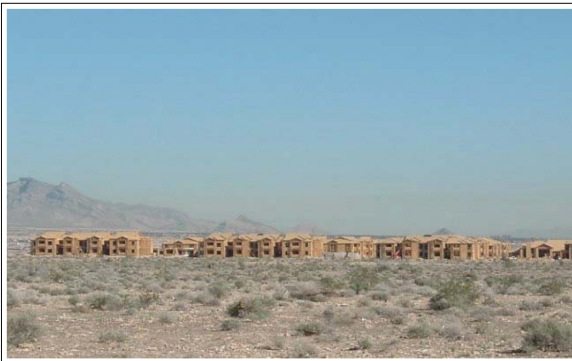
Photo 1. Wood frame homes under construction create numerous unenclosed areas where firebrands can enter and ignite. Soil disturbances associated with construction can produce excessive red brome growth in years with above normal precipitation, thus increasing the fuel hazard (Las Vegas area).
